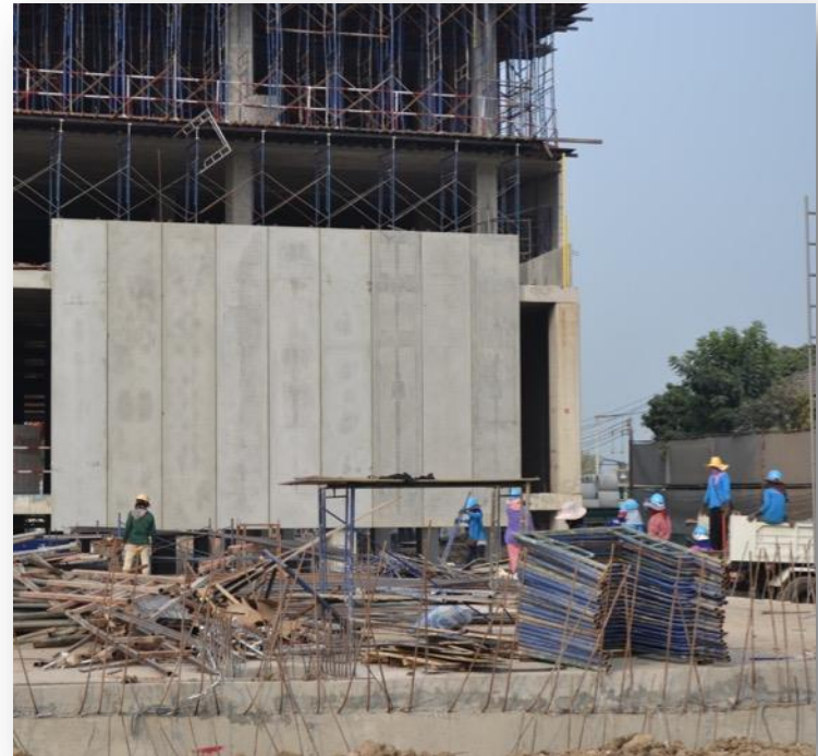
Installation Process: Series of LiteCast Panel
