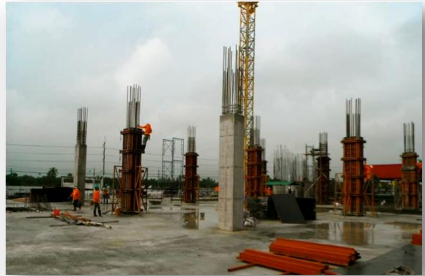
CentralPlaza Construction Site (Pillars)
