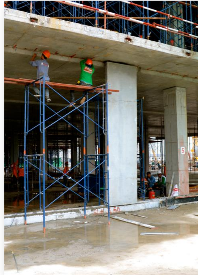
Installation Process: 1 st LiteCast Panel (Completed)
