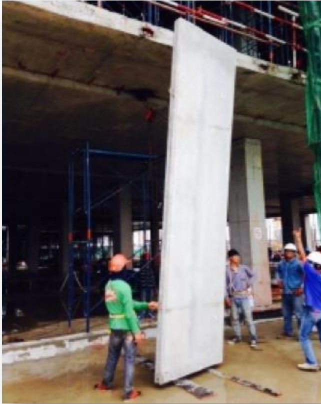
Installation Process: 1 st LiteCast Panel (During)
