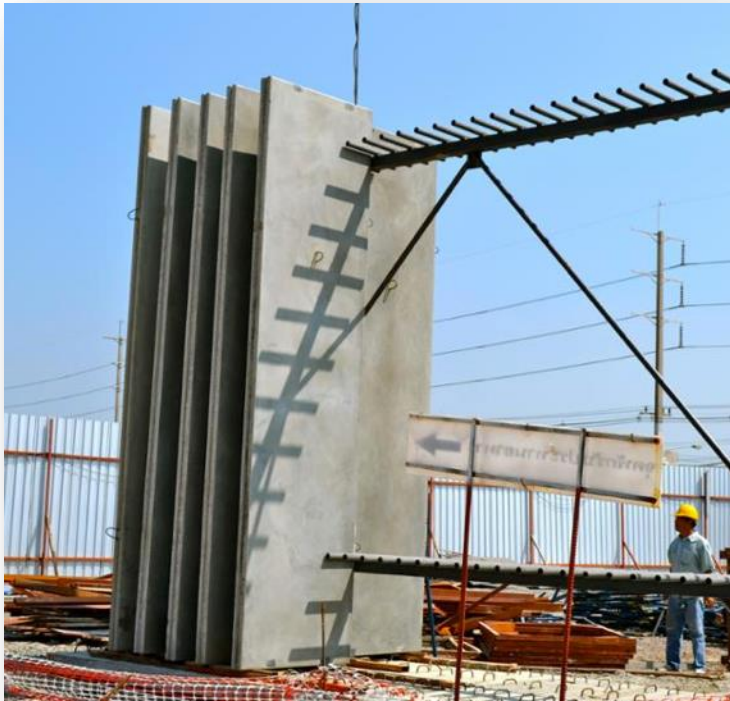
Installation Process: Series of LiteCast Panel
