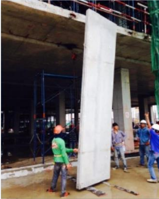
Installation Process: 1 st LiteCast Panel (During)
