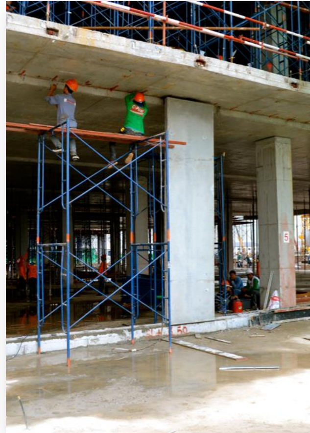
Installation Process: 1 st LiteCast Panel (Completed)
