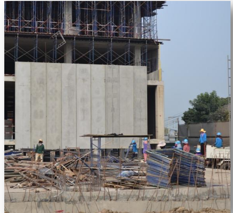
Installation Process: Series of LiteCast Panel
